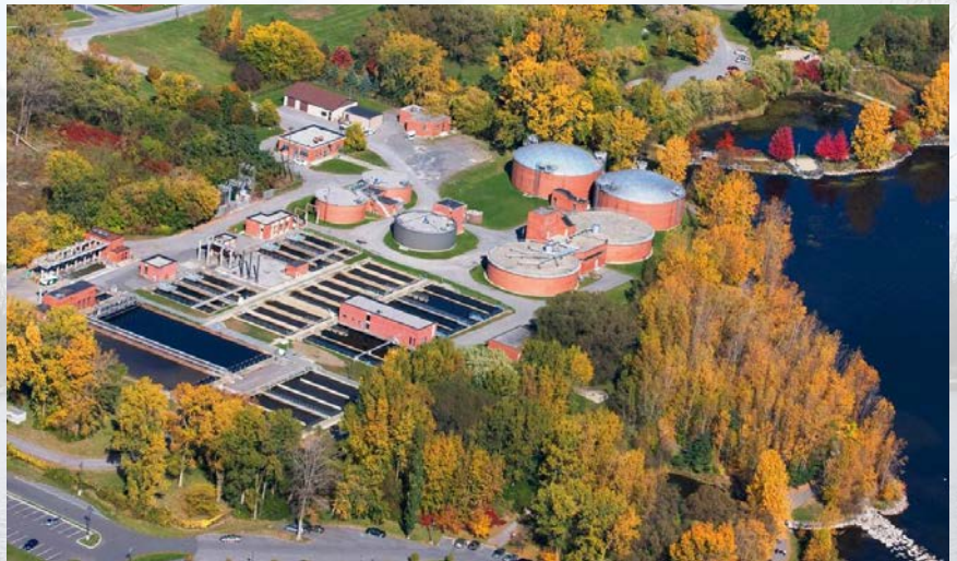
Belleville Sewage Treatment Plant
