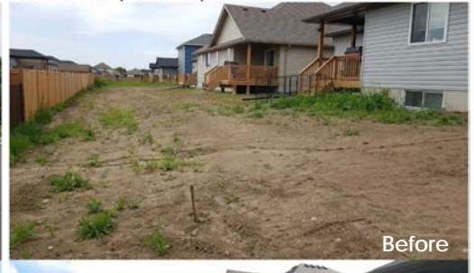
Belleville—Completed in September
